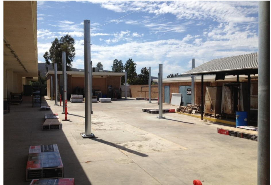
Current state of construction
